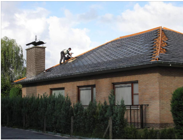
Company: Confidential Product: Sunslates 28.3 Watts Manufacturer: Atlantis Energy Model Number: Atlantis 1010 Amount: 6.99 kW Location: Prague, Czech Republic Purpose: On-grid BIPV Year: 2010
