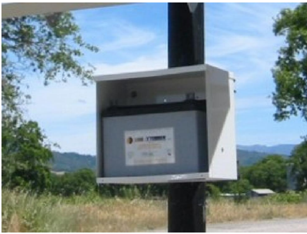
Company: Confidential Product: Battery Enclosures Manufacturer: IronRidge Model Number: LCF-01A Amount: 201 Units Location: France, Nigeria, Africa Purpose: Off-grid pole electrification Year: 2010 Project Size: N/A
