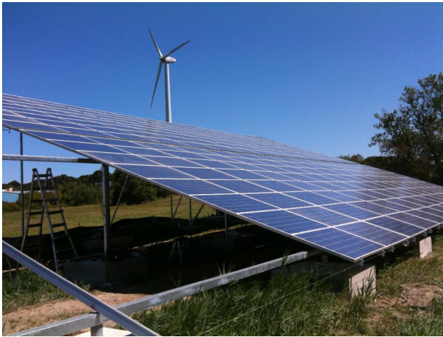
Company: Confidential Product: Moser Baer 210W Solar Module Manufacturer: Moser Baer Solar Model Number: MBPV – CAAP-200 Amount: 250kW Location: Maine, United States Purpose: On-grid Year: 2010
