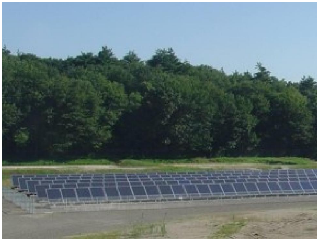
Company: United Nation Development Program Product: Ground Mounts Manufacturer: IronRidge Model Number: UNI GR-14H/04H Amount: 26.1kW Location: Beirut, Lebanon Purpose: Off-grid Ground Mounts Year: 2010
