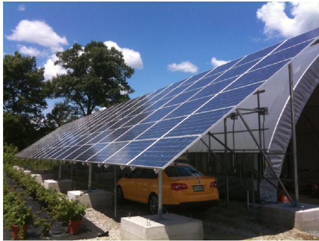
Company: Confidential Product: Moser Baer 210W Solar Module Manufacturer: Moser Baer Solar Model MBPV – CAAP-200 Amount: 150kW Location: Vermont, United States Purpose: On-grid Year: 2009
